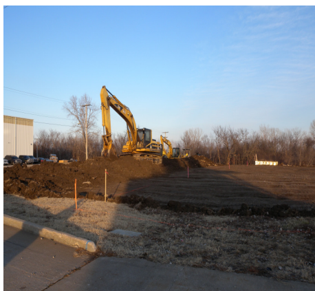
Construction on Tulsa's new Paint Shop
